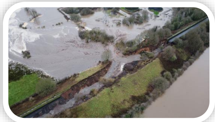
Bridgewater Canal collapse (photo courtesy Inlands Waterway Association)
