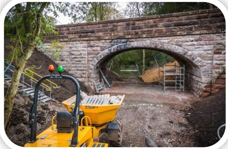
Great Musgrave Bridge after removal of concrete infilling (photo courtesy New Civil Engineer)
