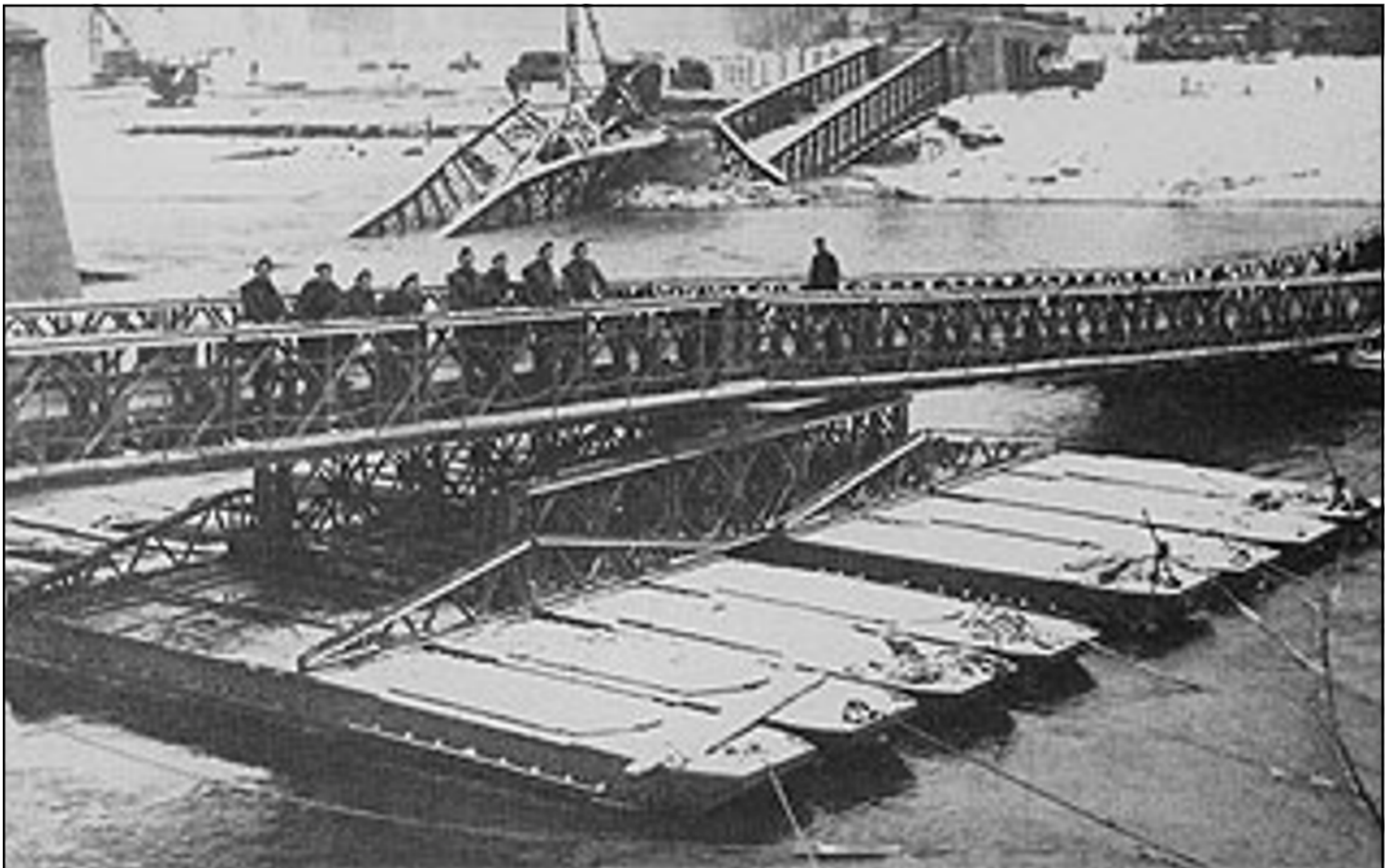
Class 40 Bailey Pontoon Bridge built over the river Meuse at Maeseyck by VIII Corps Troops Engineers January 1945
