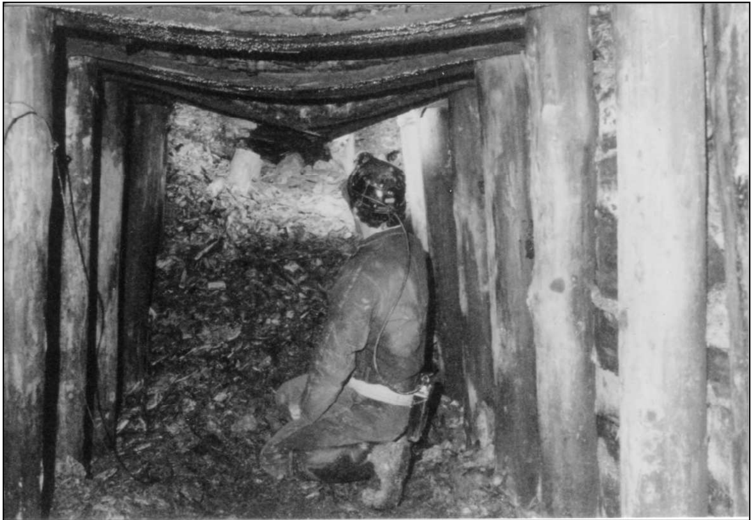
The collapsed roof and timbers near the end of the accessible part of the incline in 1984
