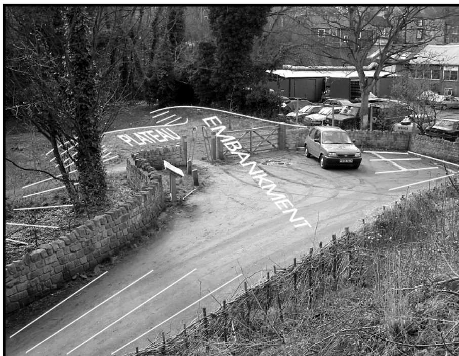
Earthwork at Mill Lane, Dronfield.
